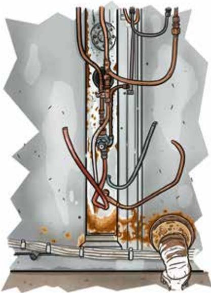
Fig. 11: Inadequate hygiene on a humidifier
